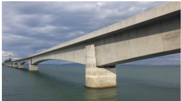
写真-5 橋梁の排水溝外
